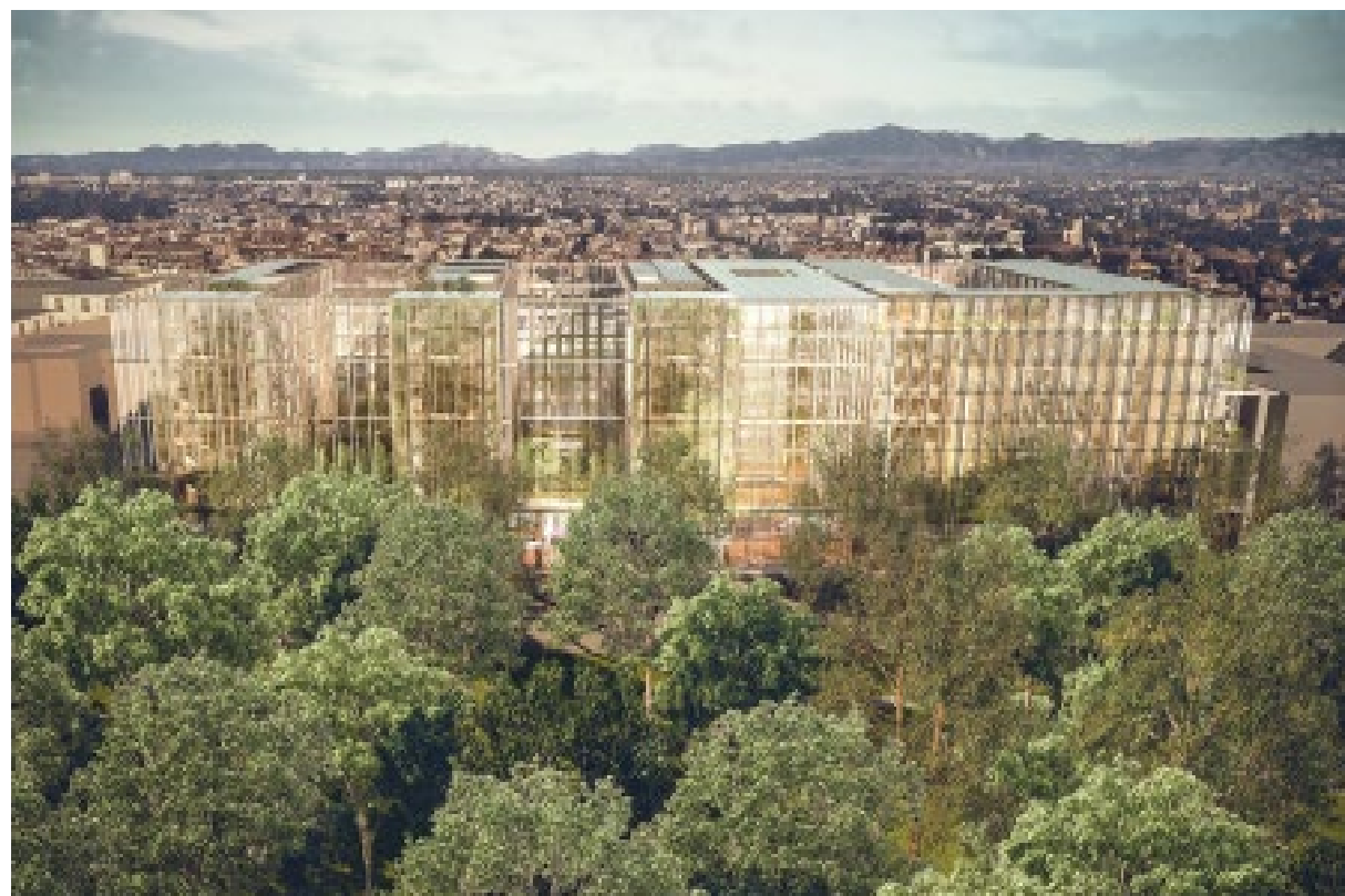
ENEL HEADQUARTERS ROME
